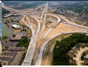
Interstate 465 Reconstruction, Indiana
